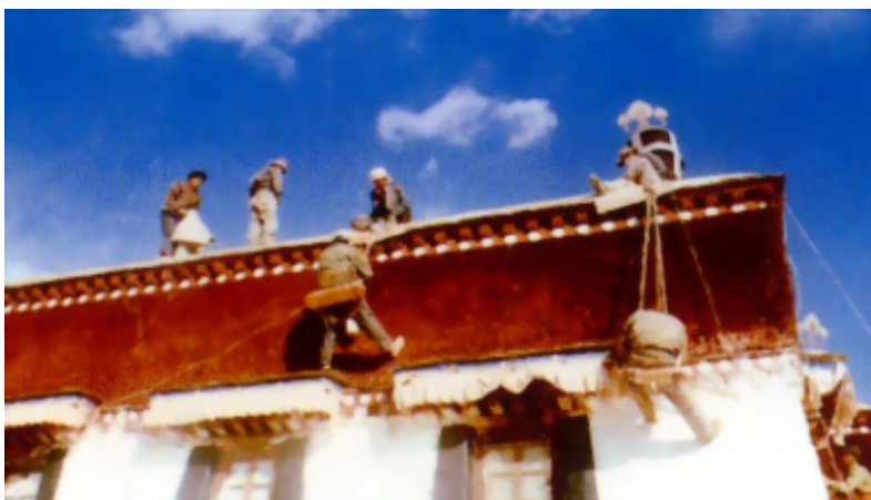
Yearly application of earthen materials outside the walls of the Potala Palace
